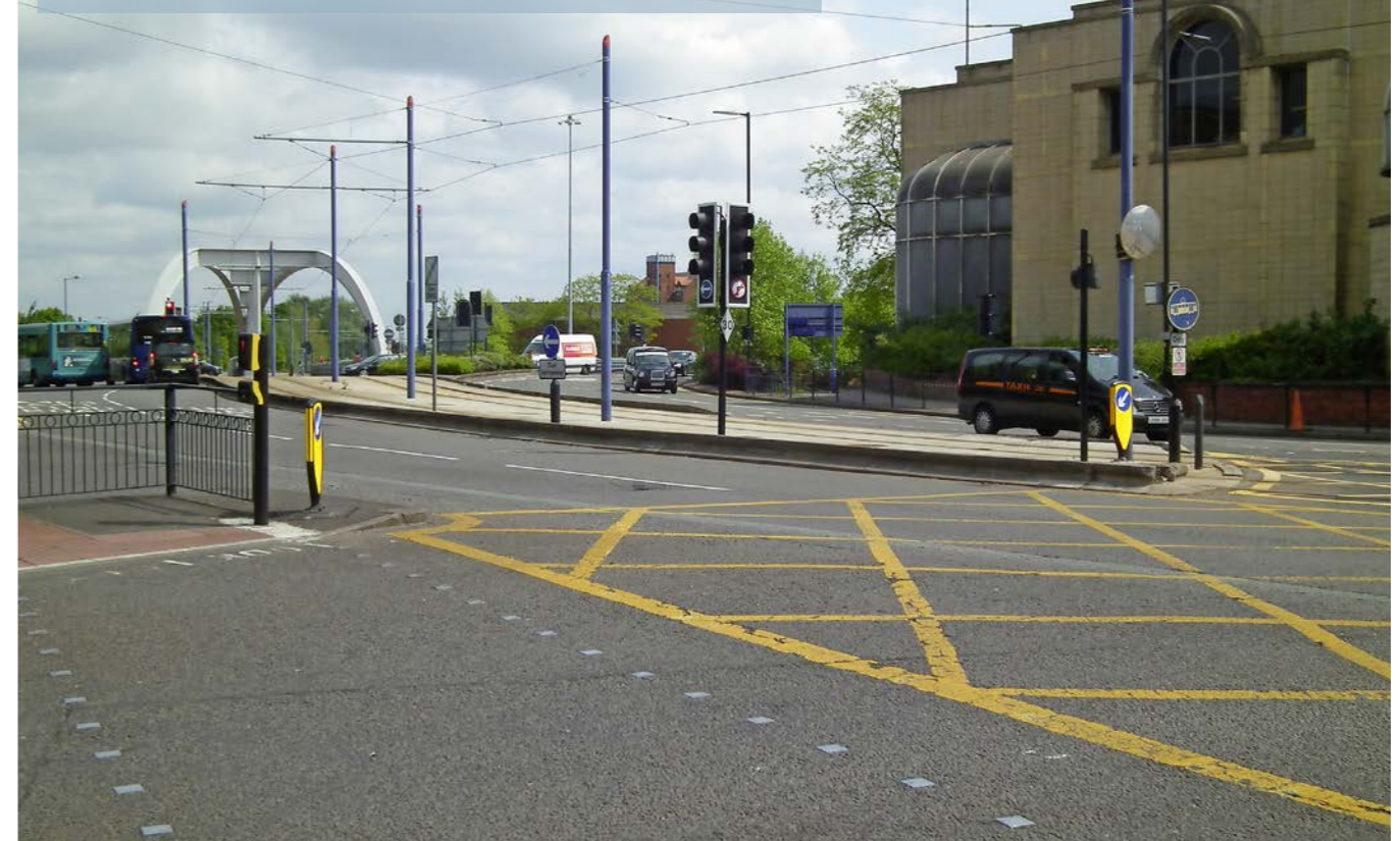
The site of the future junction of the Wolverhampton Station extension with the existing line to the St George's terminus, as seen looking south east from the junction of Pipers Row and Bilston Street on May 30 2016, with the distinctive Bilston Street Island tramway bridge in left background. MIKE HADDON.
