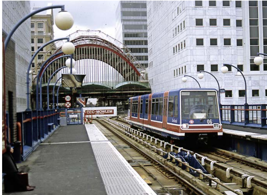
Canary Wharf station is pictured on December 6 1991, less than a month since opening. The six-platform station was not ready in time for the DLR's official opening in August 1987, after it was realised that demand had been considerably underestimated and station plans would have to be revised. COLOUR RAIL.
