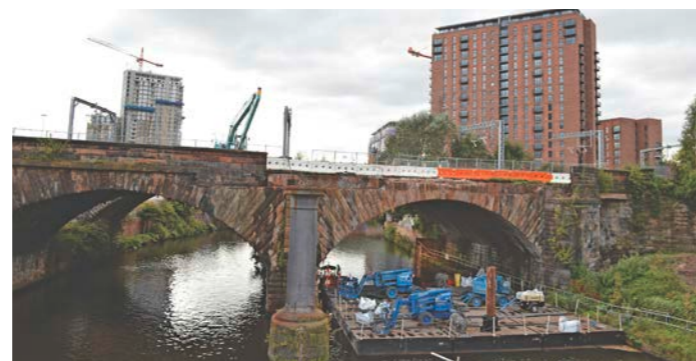
▲ The 63ft span of George Stephenson's Grade I-listed bridge over the River Irwell, built in 1830, has been revealed to full public view by Network Rail for the first time in more than 150 years. PAUL STEPHEN.
