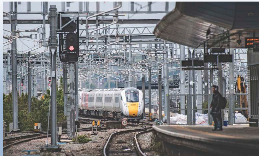
▲ IP delivered more than £6 billion worth of work in the last financial year including on the Great Western Route Modernisation. An Intercity Express Programme test train approaches Reading on April 29 beneath newly erected overhead line equipment, which will be energised next year. JACK BOSKETT/RAIL.
