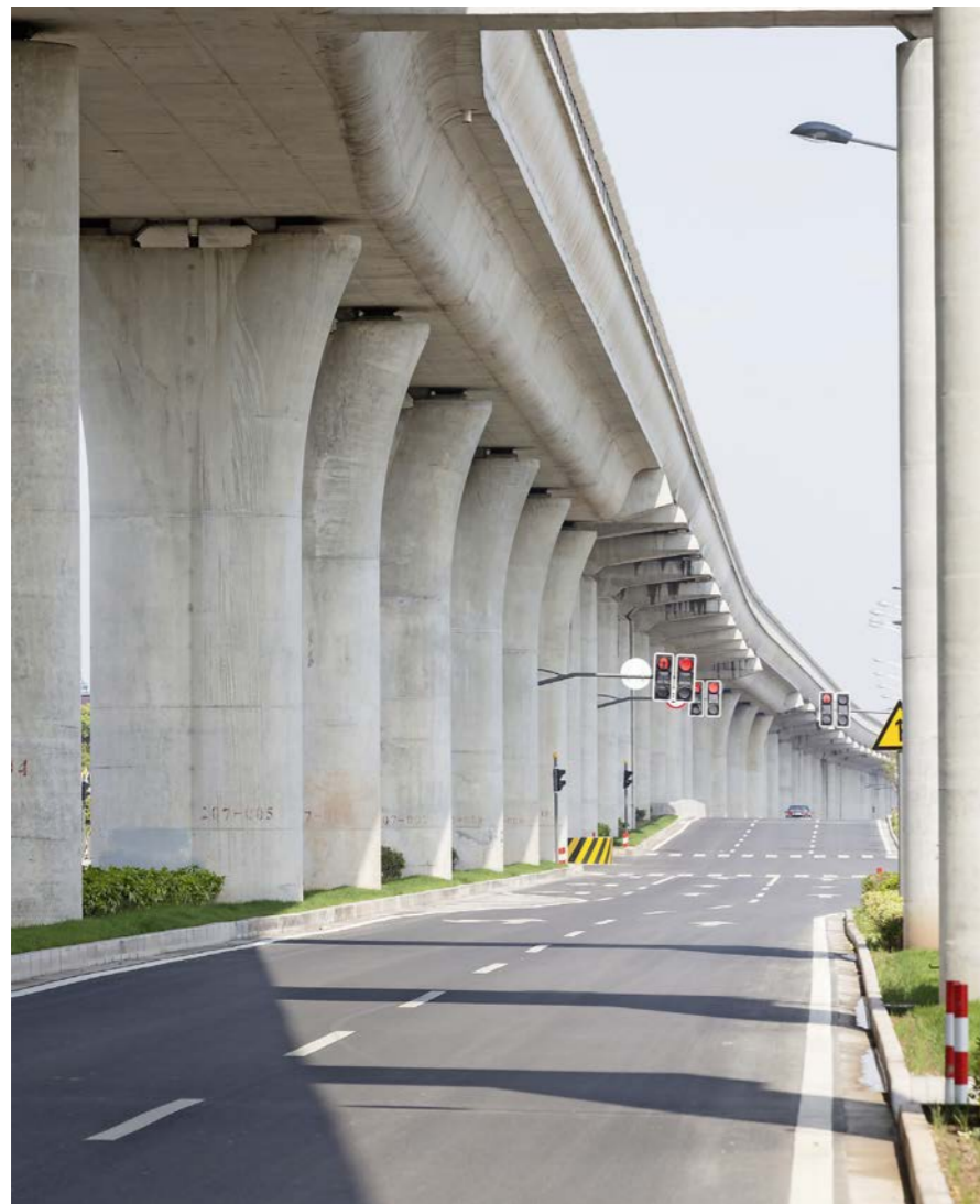
More than 450km of SYSTRA-developed U-shaped viaduct has been designed and built since 1992. The world's longest metro line in Shanghai includes 45km of a highly cost-efficient, time-saving construction solution, as pictured here. P. WACK/CAPA/SYSTRA.
