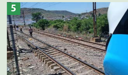
5. Taken at Piensaarspoort station, members of the public are able to access the tracks through damaged fencing and gaps in the boundaries.
