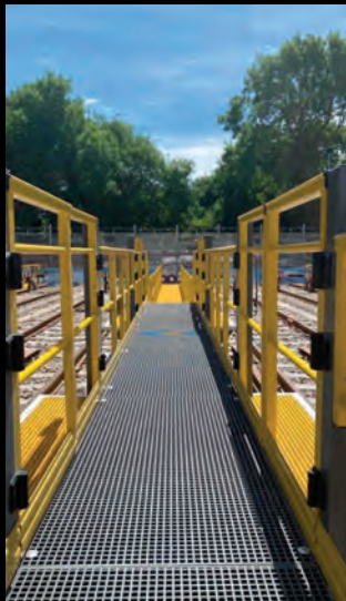
Driver Access Platforms
